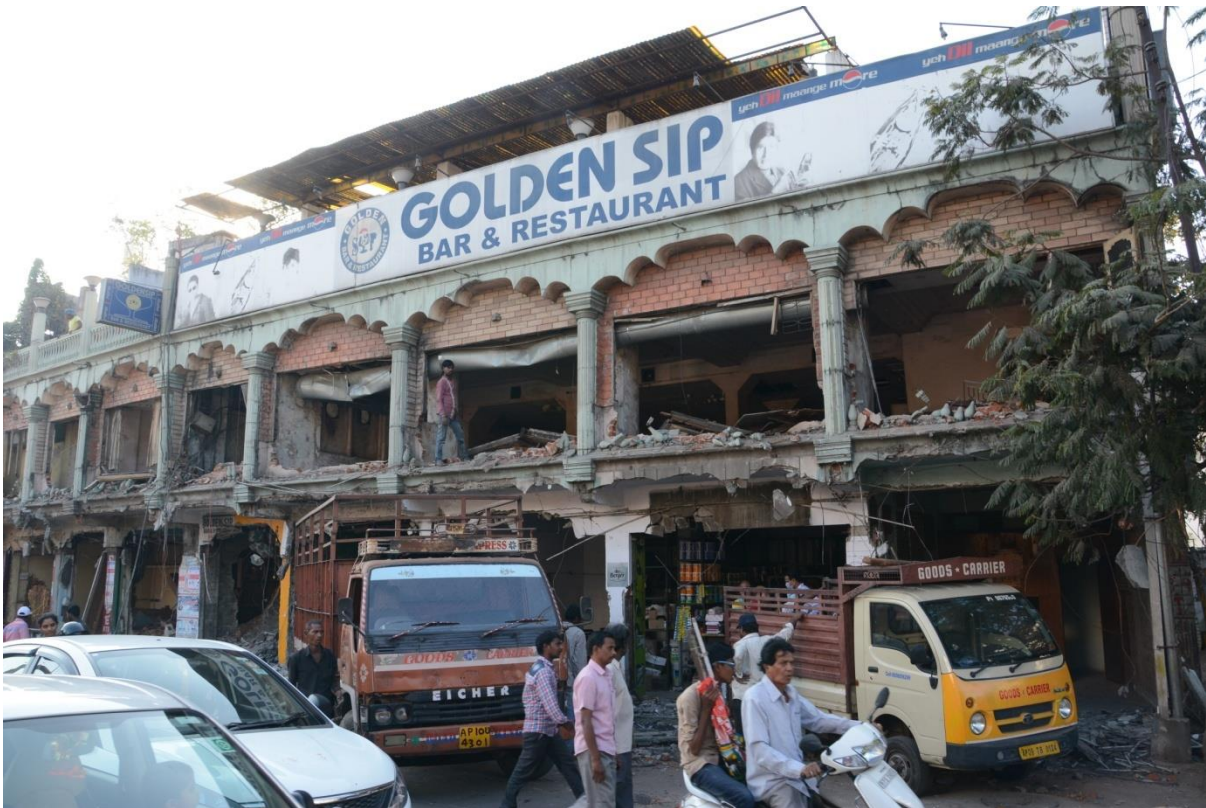
Dismantling of Golden Sip Hotel in progress at Musheerabad junction on Metro Rail Corridor II on Saturday (January 21, 2017)
