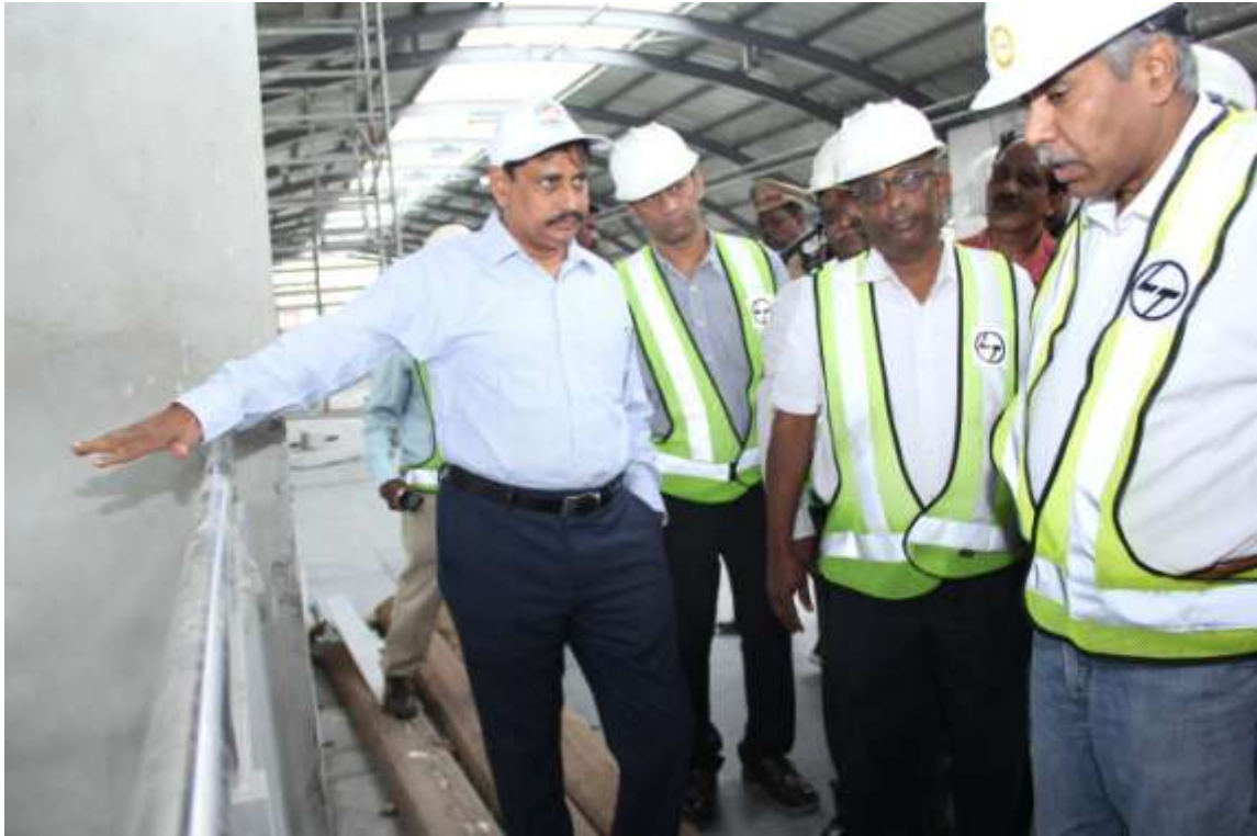
MD, HMRL Mr. NVS Reddy inspecting rain water drainage arrangements on Metro Rail viaduct between Madhapur and Hitec city Metro stations along with MD, L&TMRHL Mr. Shivanand Nimbargi on Saturday (26.08.2017)
