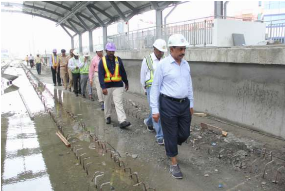
MD, HMRL Mr. NVS Reddy inspecting the rain water drainage arrangements on Metro Rail viaduct between Prakashnagar and Parade Grounds Metro stations MD, L&TMRHL Mr. Shivanand Nimbargi on Saturday (26.08.2017)
