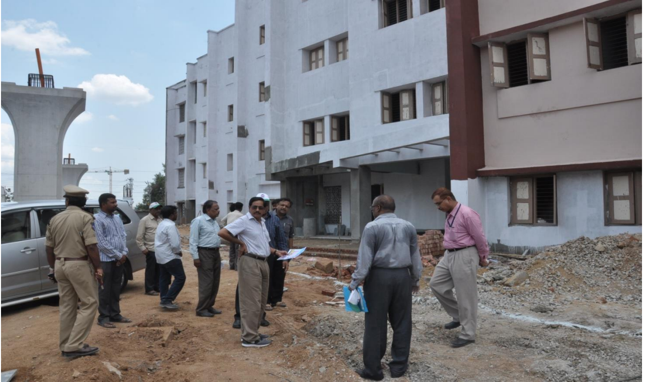
MD, HMR Mr. NVS Reddy inspecting Government School complex at Chaderghat, being built by Hyderabad Metro Rail on June 11, 2015
