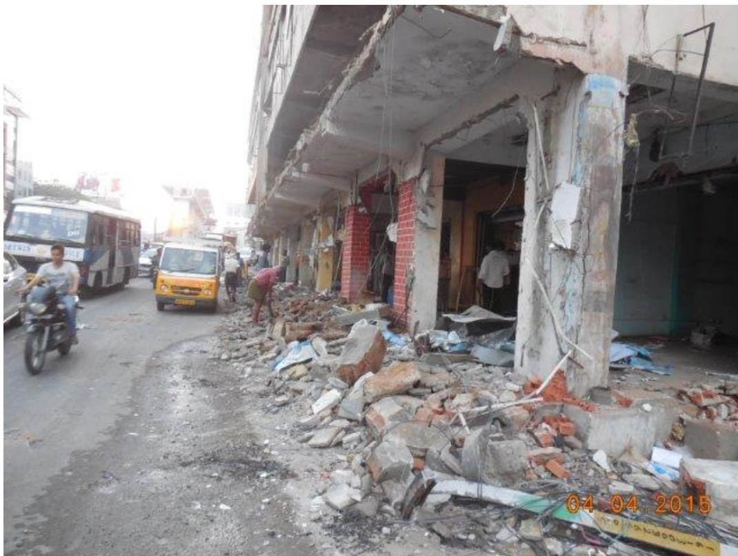
Dismantling of Jabbar building in progress at Begumpet
