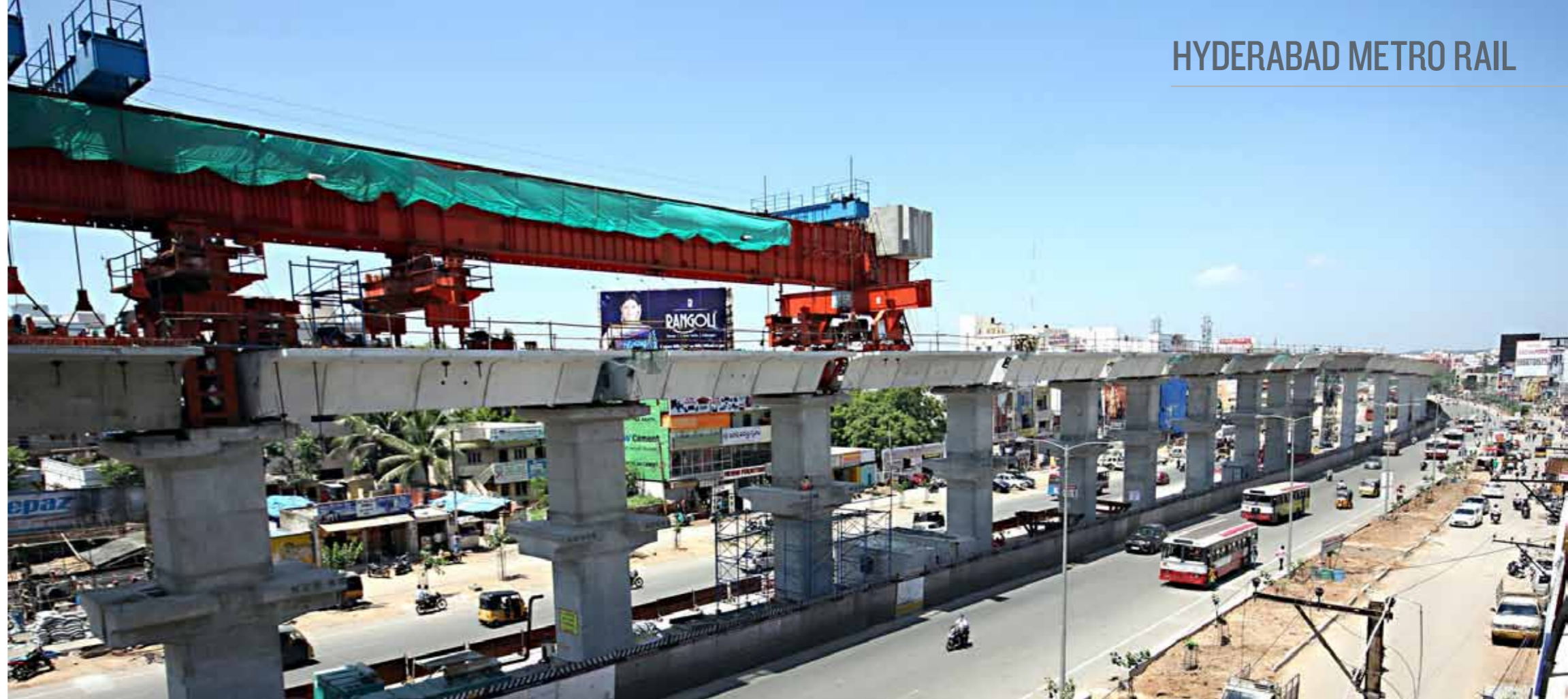
Launching Girder – State of the art construction equipment used to build elevated viaducts of Hyderabad Metro Rail
